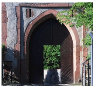
Gate of the gate-tower
