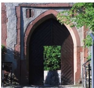
Gate of the gate-tower
